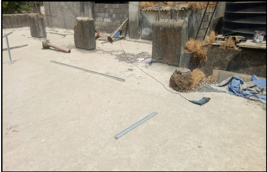
Before Installation of solar panel on terrace
