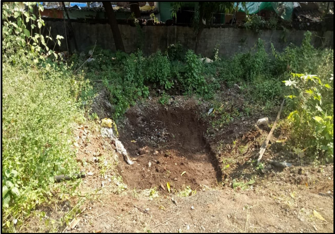
Compost pit in prelim stage
