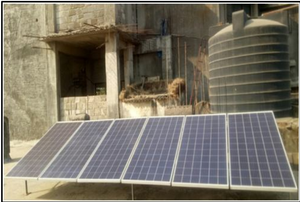
Installation of solar panel on terrace
