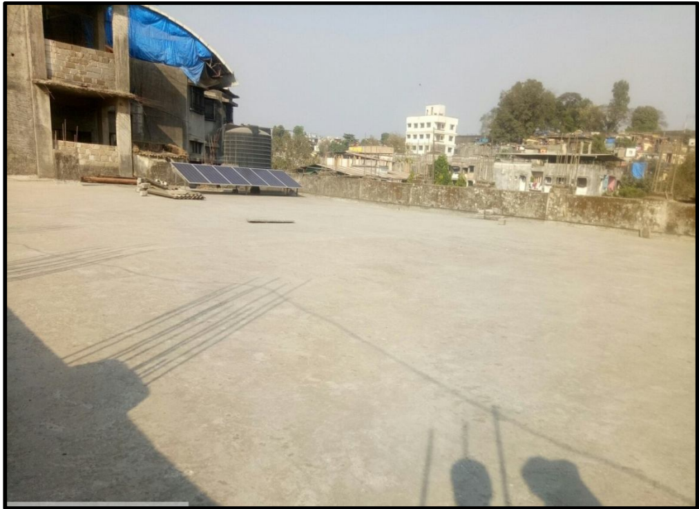
Installation of solar panel on terrace
