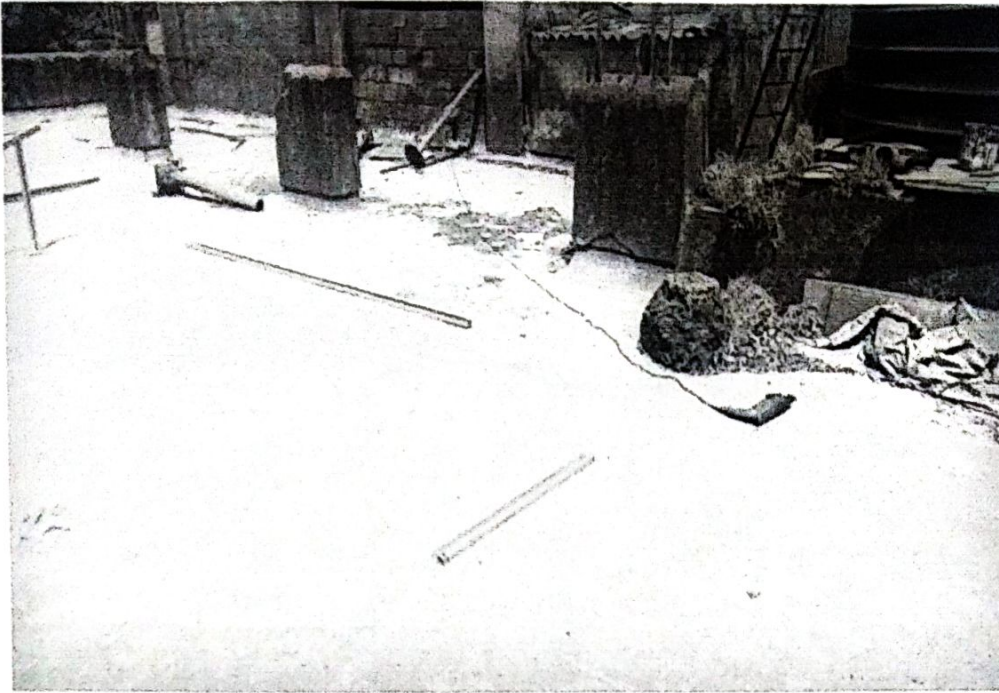
Before installation of solar panel in college on terrace
