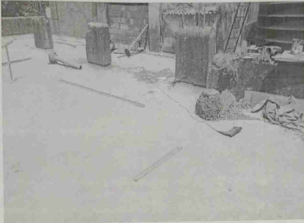
Before installation of solar panel in college on terrace
