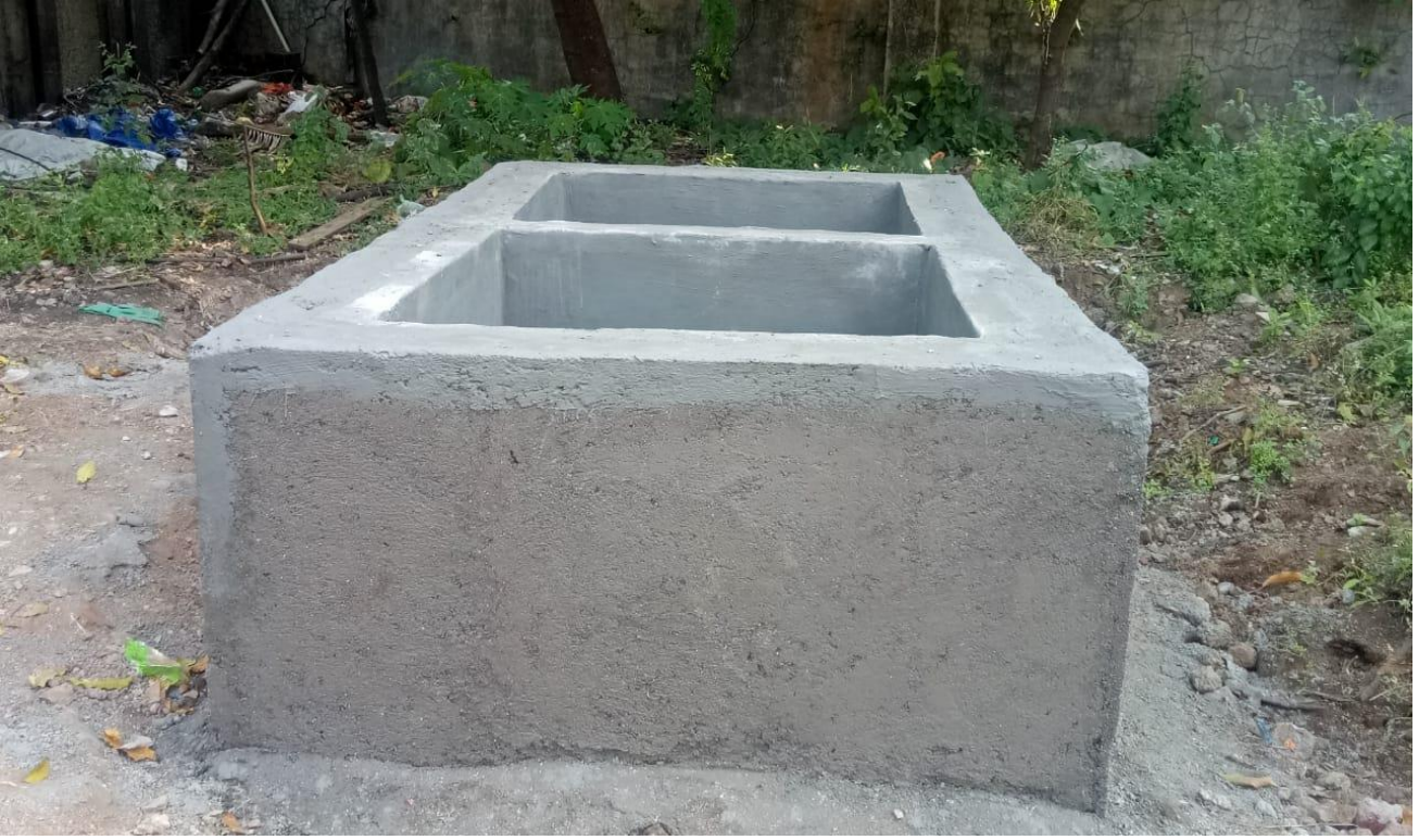
Compost Pit For Litter In School Side
