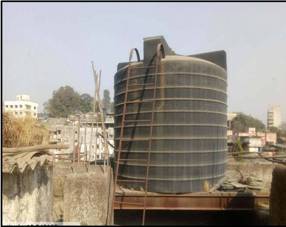
Water storage tank
