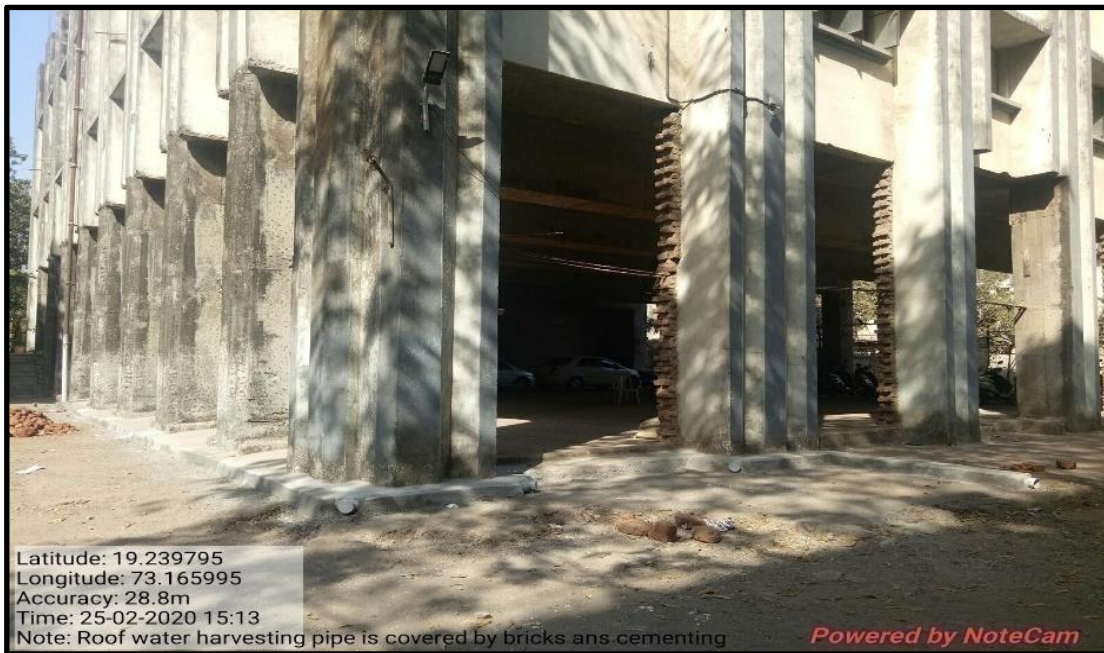
Collection Harvesting water pipeline
