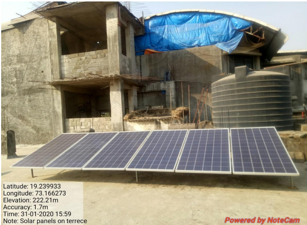
Installation of solar on terrace
