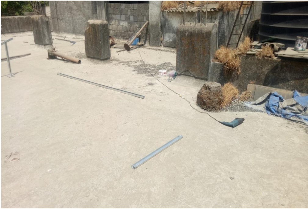
Before installation of solar panel in college on terrace
