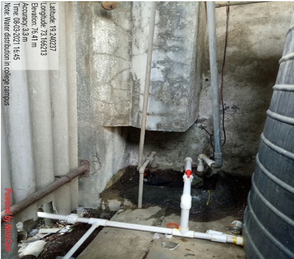
Open well water storage in a tank and distribute in college campus
