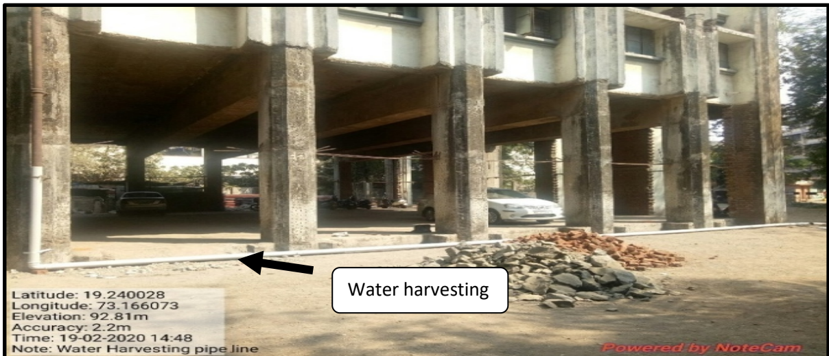
Collection Harvesting water pipeline
