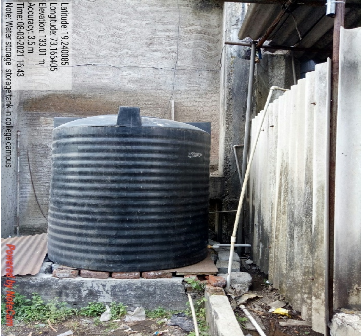
Water Storage tank
