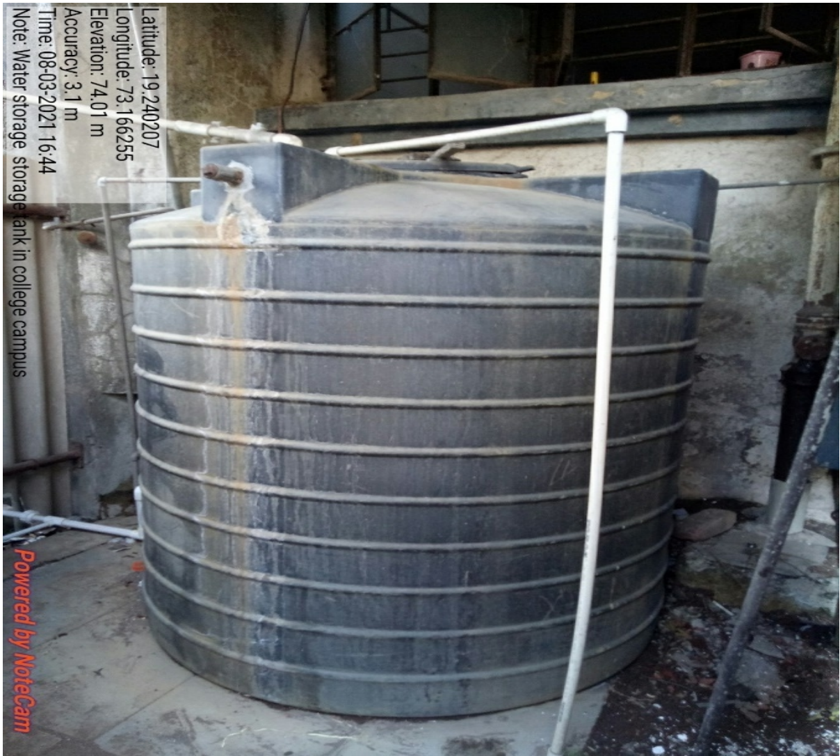
Water storage Tank
