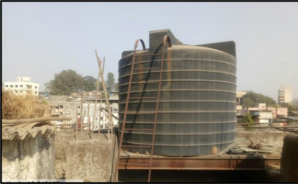
Water storage tank
