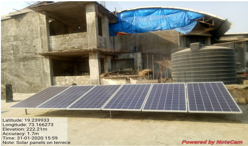
Installation of solar on terrace
