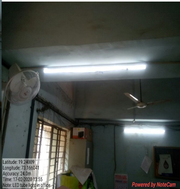
LED Tube light used office
