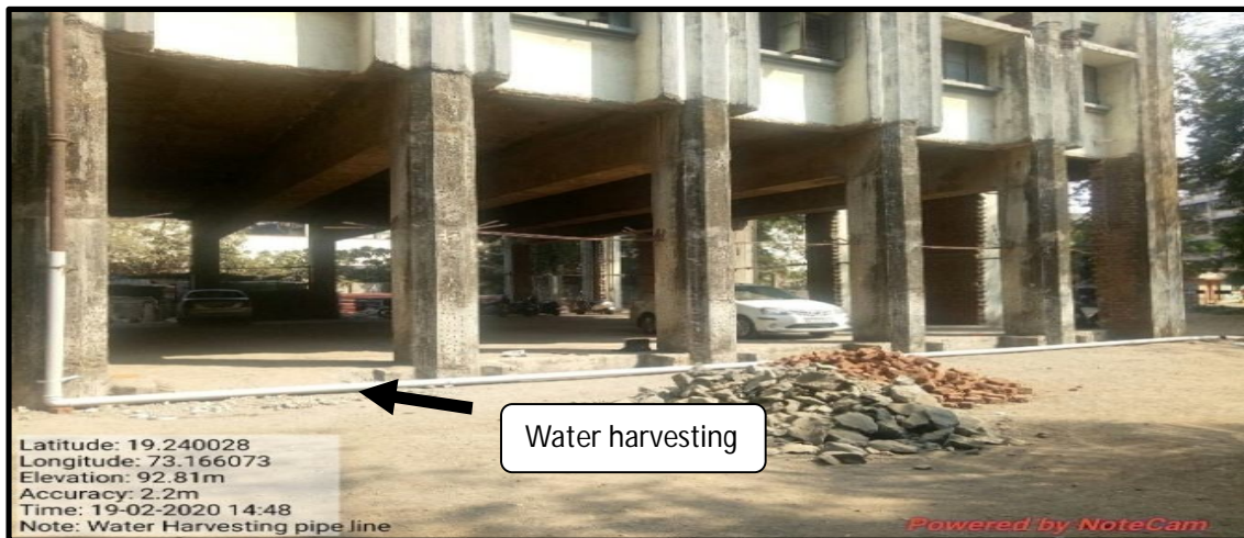
Collection Harvesting water pipeline
