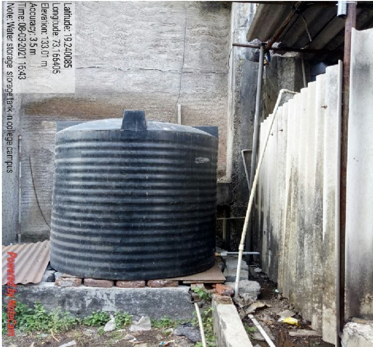
Water Storage tank
