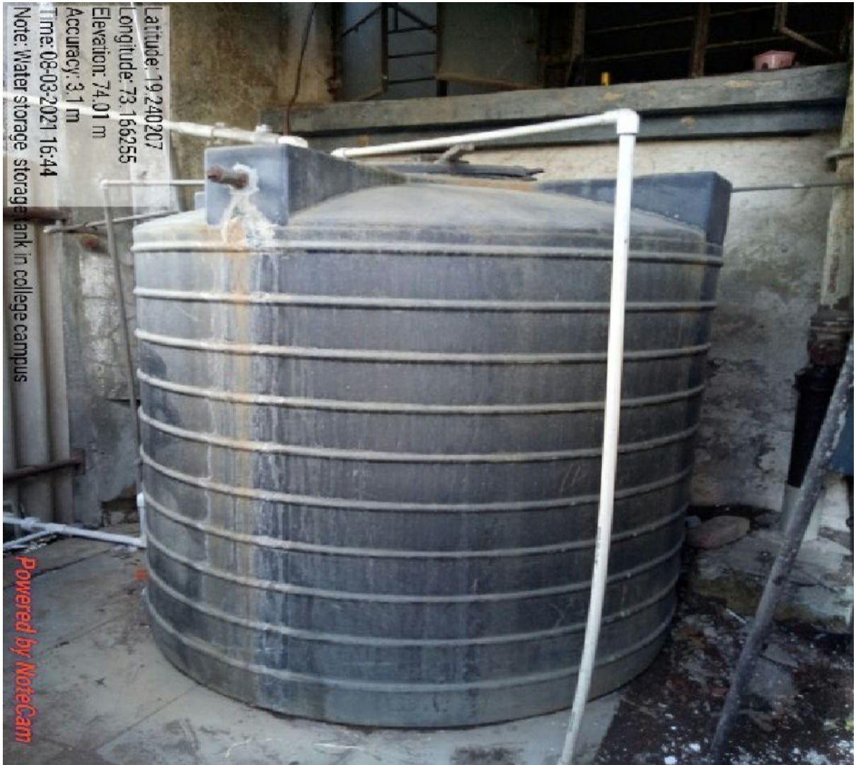
Water storage Tank
