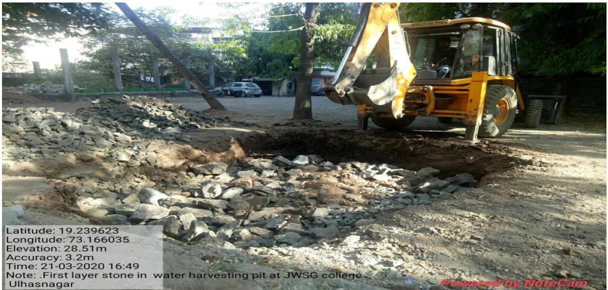
First layer of stones dumped in water harvesting pit
