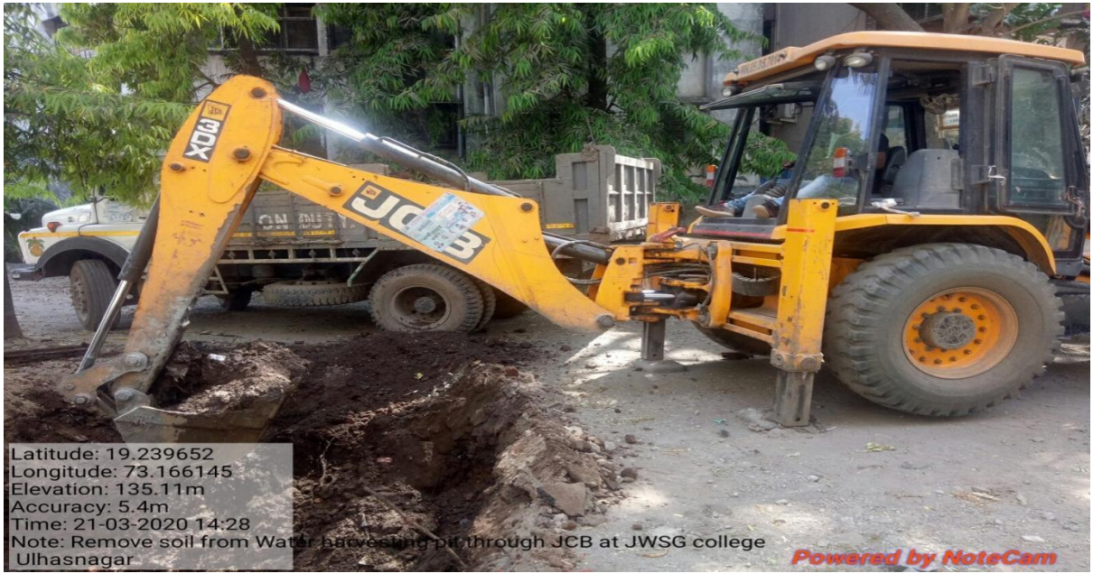
Soil removes from water harvesting pit through JCB in college campus
